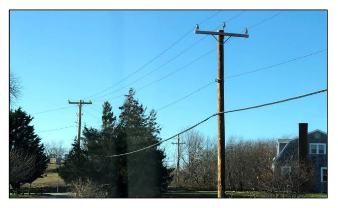
The New Harbor Circuit is being rebuilt with all new poles and larger conductor. The project is 80% complete. The new line is constructed for a Wye configuration and is ready for our voltage conversion.
