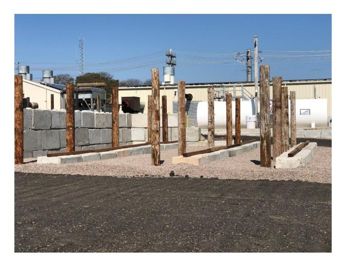
BIUD recently completed a new pole yard that meets best industry practices for storing wood poles treated with penta-chlorophenol. These storage bunks improve the employee safety aspect of loading/off-loading poles, relocates the poles away from a Class I wetland buffer and improves the "road appeal" from Beach Avenue. This latest project is a continuation of our work towards cleaning up the facility, making full use of the property and improving the workplace for our employees.
