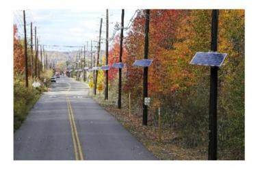
The pole attached solar units are comprised of a solar panel, micro-inverter and communication module mounted on a patented racking system. A two-person crew installs the solar units, which connect directly into the PSE&G power grid that serves homes and business.
