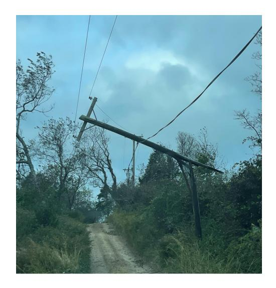
On Wednesday October 23<sup>rd</sup>, the season's first nor'easter impacted Block Island. The high gust was 87 mph. The 24-hour event caused four separate line section outages that affected roughly 100 members. Crews had to replace three broken poles like this one shown on Corn Neck.
