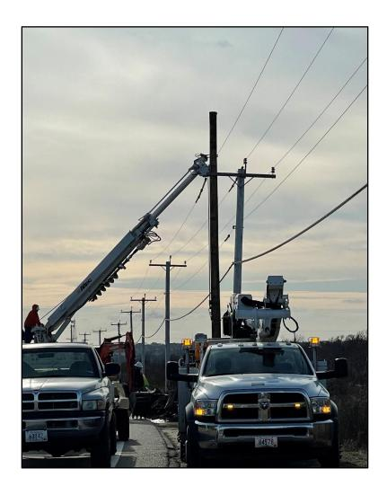
The Voltage Conversion project is underway and will start to generate questions from our members. The poles recently set on Corn Neck and Center Road are ten feet taller than our normal poles to provide space necessary for the step transformers and fuses. These poles serve as a visible boundary to where the converted wye system will end on each circuit. These will be relocated in future project phases and eventually removed.
