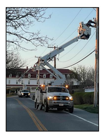
Phase One of the Voltage Conversion project is complete. Crews worked during early morning hours on two separate days rewiring and converting more than 100 transformers without incident. We estimate that approximately 60% of our summertime load has been converted to 4,160 WYE. This will improve power quality, voltage and relief several overloads all of which will help reduce system losses.
