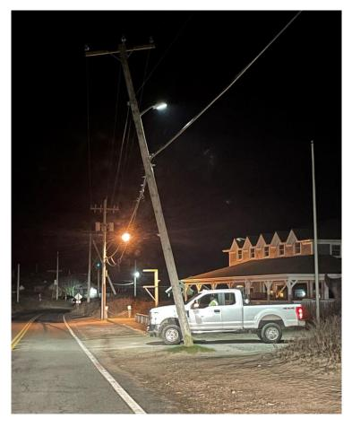
When it rains it pours. This picture was taken the night that the island was being powered by diesel engines after the submarine cable tripped. At approximately 10 PM, while we were working with RI Energy to test the submarine cable, we got the report of this broken pole in front of the Beachhead. Although BIUD has dramatically improved reliability by changing roughly 600 poles in the past five years, we still have a lot of work to do to rebuild our pole plant.
