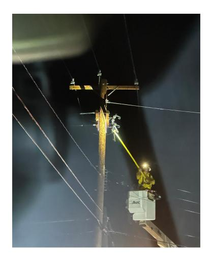
Lead line worker Evan Carey reenergizes the Mitchel Lane tap following a line fault caused by a downed tree behind the Quankenbush residence. On the evening of January 10, 2024, a power storm subjected Block Island to heavy rain and wind gusts > 80 mph. Three separate outages, affecting roughly 100 members, were all caused by high winds. Two of the three were caused by falling trees.
