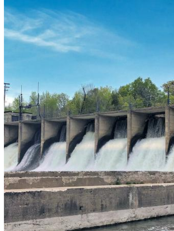
Turner Falls Hydro Montague, MA
